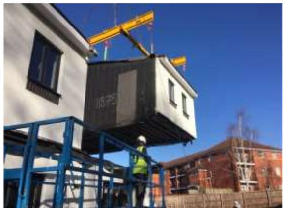
This scheme uses the Ilke Homes modular housing system ([www.ilkehomes.co.uk](http://www.ilkehomes.co.uk)). Homes are built to exacting standards in a precision engineering factory in Knaresbrough, Yorkshire, before being craned into position on site. We have halved the amount of concrete (a huge generator of CO2) used in the foundations compared to a typical new house. This is a true 'modern method of construction' (MMC) system.
